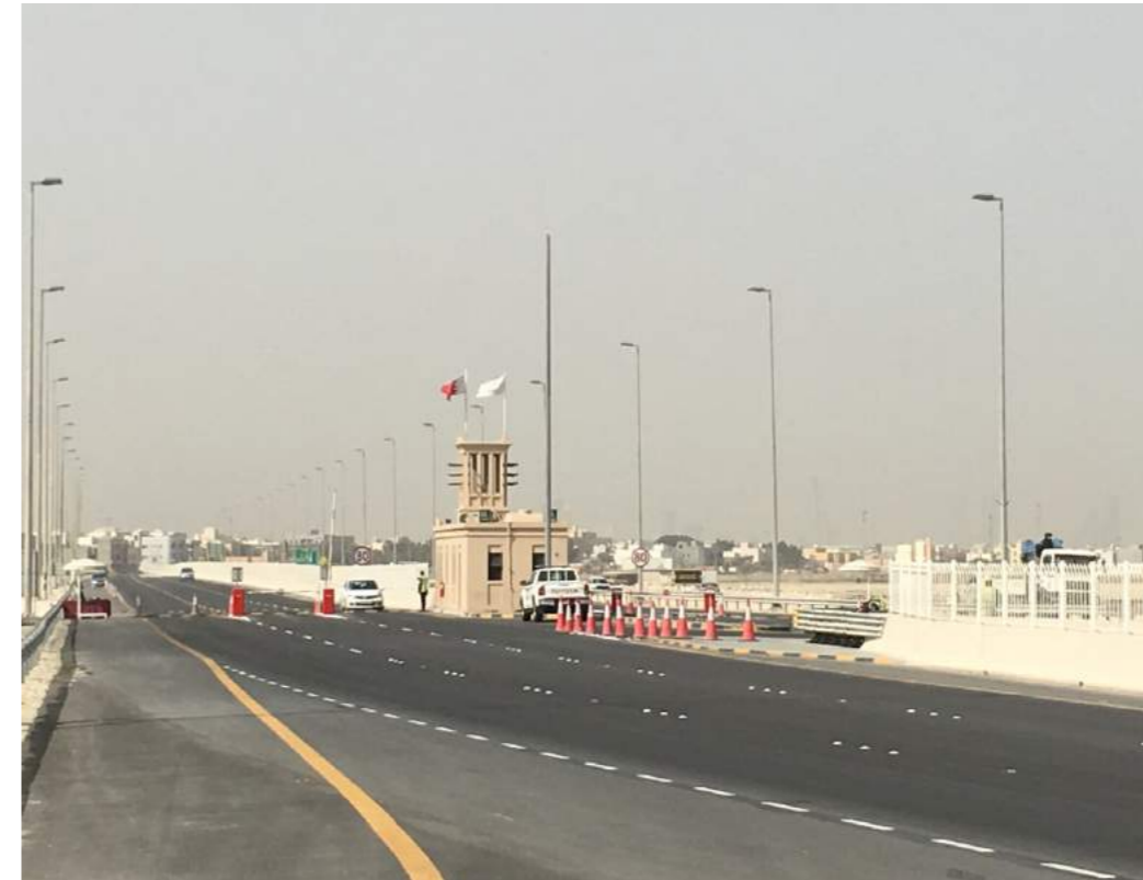
Figure 2.16: Diyar Al Muharraq Site Access Gate
